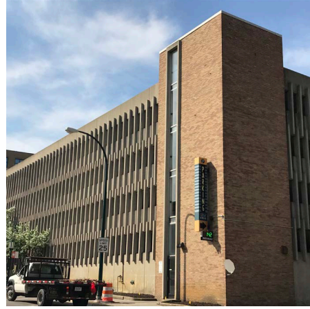
Left: Current North Old Woodward parking deck.
